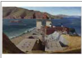
5773 Golden Gate Bridge Ray Strong
